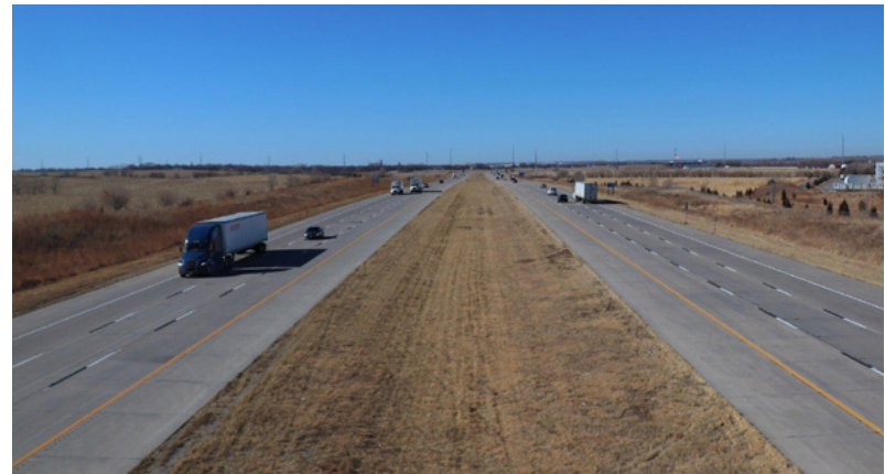
Interstate 80 near Waverly, looking west from the 134th Street bridge. The pictured area would change significantly if the long-discussed East Beltway comes to fruition, as the beltway would connect with I-80 and U.S. 6. - Sam Crisler, The Waverly News
