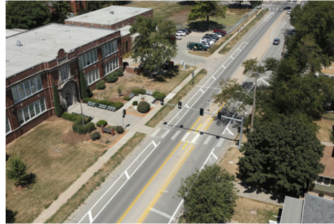
Implementation Award Recipient Saratoga Elementary Safety Implementation Project
